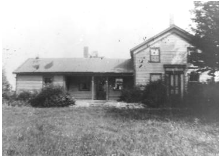
This farmhouse stood on the Shanahan property in Java, NY. It was the first property purchased for what would become the Beaver Meadow Audubon Center. Today, visitors can see the foundation of this house while hiking on the Old Homestead Trail.
